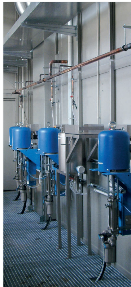
Plant construction and installation
